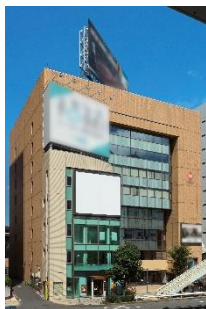
Kita Aoyama Building
