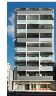
Cross Residence Kiyosumi-Shirakawa (Koto-ku, Tokyo)
