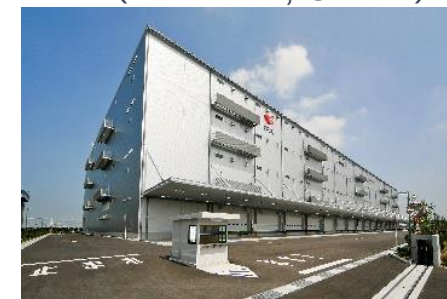
Sakai Logistics Center North Building (Sakai-shi, Osaka)
