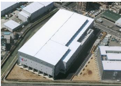
Toda Logistics Center (Toda-shi, Saitama)
