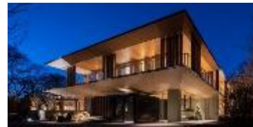
ØST Residence Karuizawa
