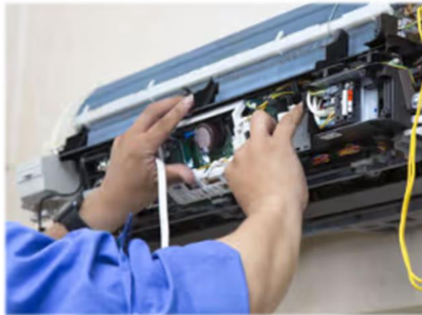
<Air conditioner installation>
