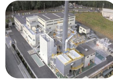
Fujinomiya Business Office (incineration)
