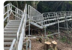
Temporary construction equipment (Other Business)
