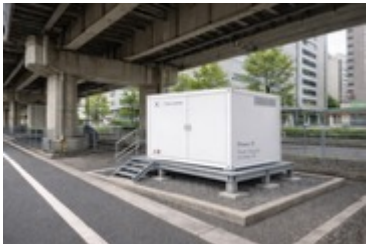
Areas under elevated tracks
