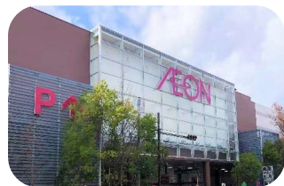
Exterior wall painting
