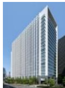
ARK Hills South Tower
