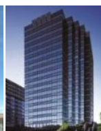
Koraku Mori Building
